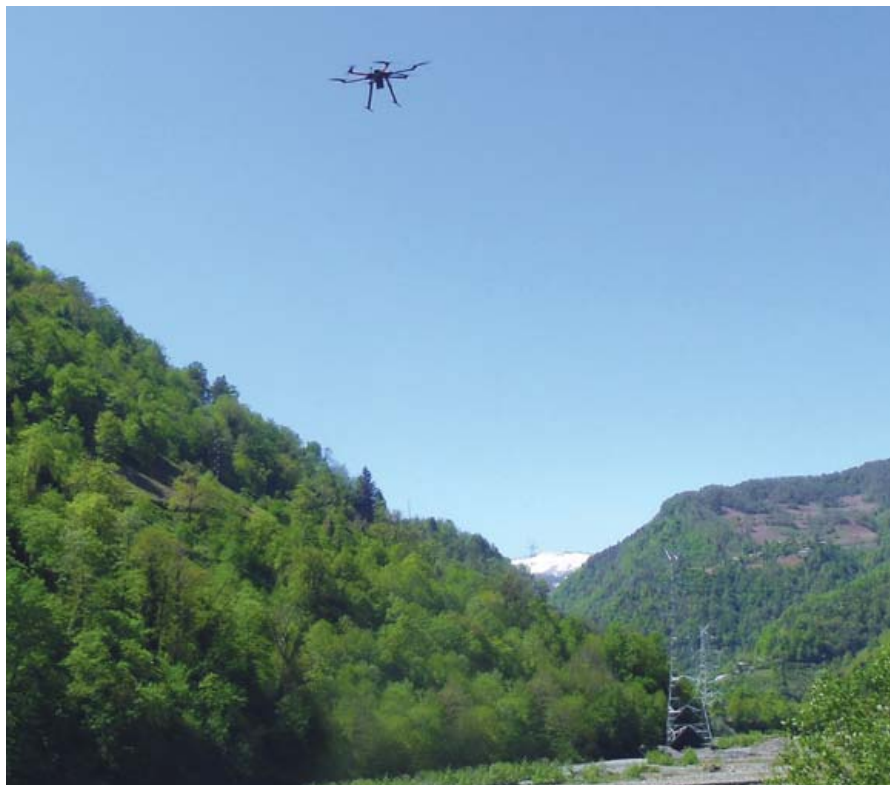
▶ Stringing Using Drone at Project Site in Georgia
