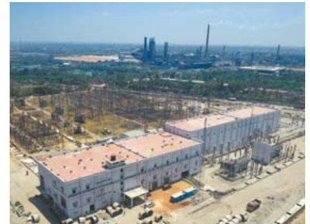
▶ 400/220/110 kV GIS Substation and 400/220/110 kV Cabling at Manali, Tamil Nadu, India
