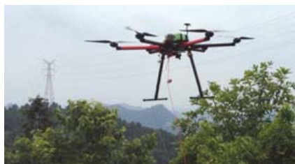
▶ Use of Drone for Stringing
