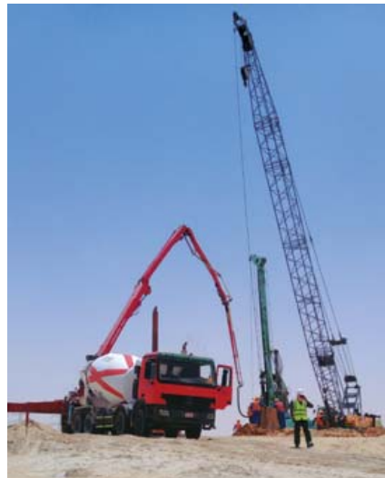
► Pile Foundation Construction in progress in the Desert in Abu Dhabi
