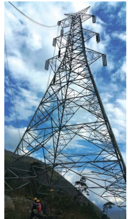
▶ 400 kV Transmission Line in Bhutan
