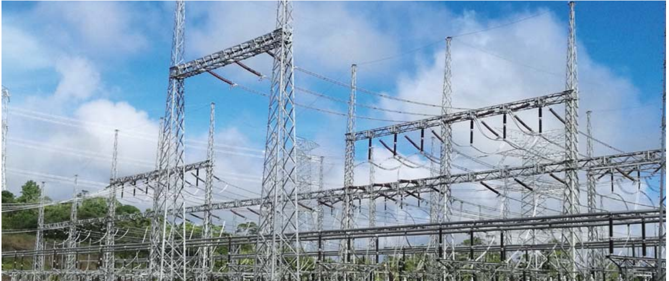
▶ 275 kV Substation Project in Malaysia
