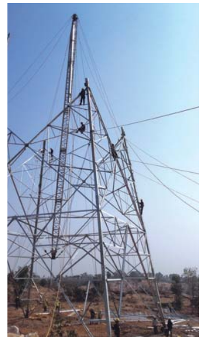
► Use of Gin Poles for Tower Erection
