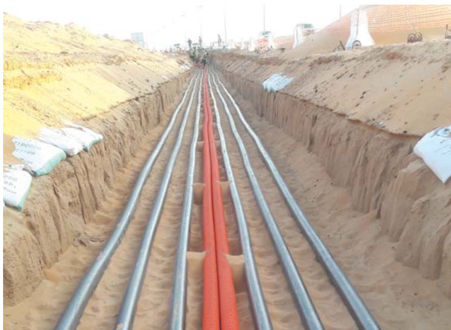
► Cabling Works associated with 132 kV Transmission Line Project in Sharurah
