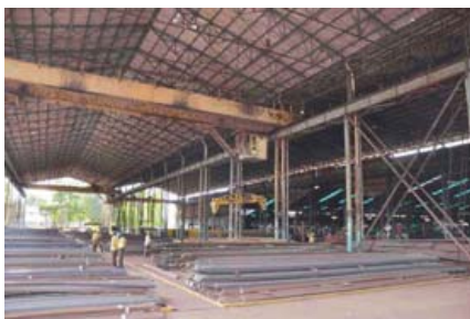
▶ Tower Manufacturing Factory, Jabalpur, Madhya Pradesh, India
