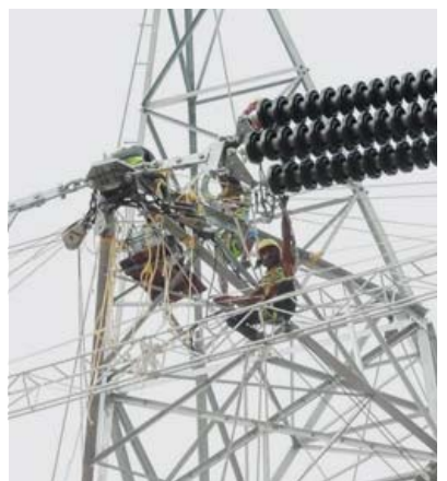
► Stringing using Sag Bridges
