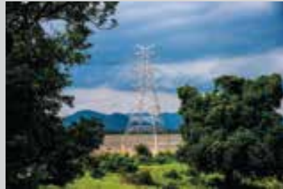
765 kV Transmission Line from Srikakulam to Angul, Odisha, India
