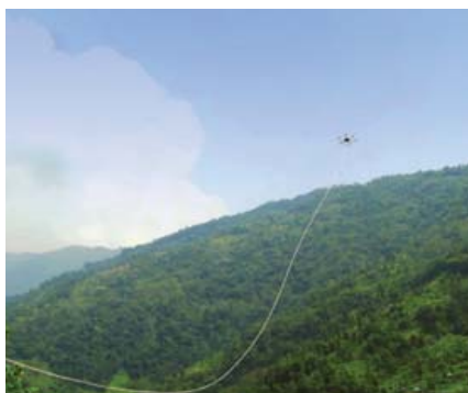
▶ Stringing Using Drone for a Project in Sikkim, India
