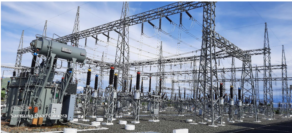
132 kV Air Insulated Substation, Papua New Guinea
